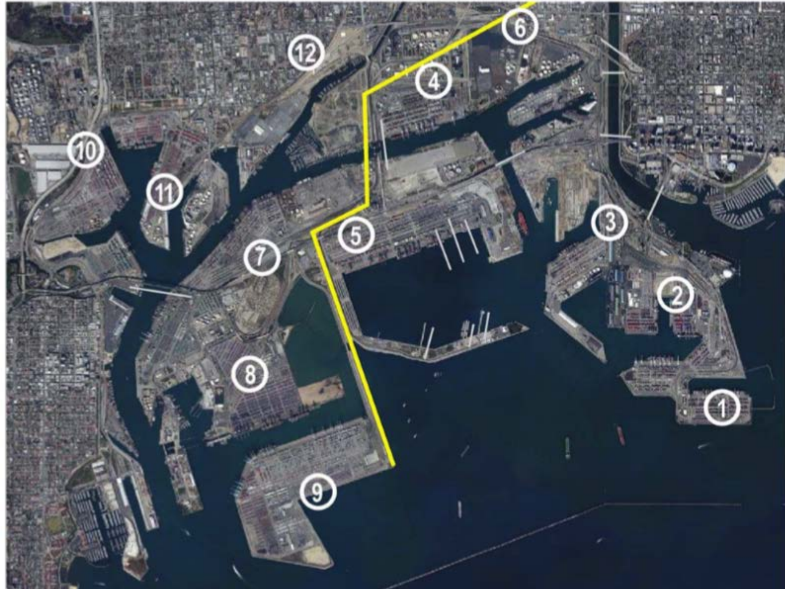
Figure 14.300 On-Dock and Support Rail Yards in San Pedro Bay
