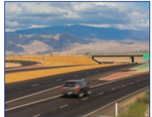
Traffic exits State Route 178 at the newly completed Morning Drive Interchange in Bakersfield.
