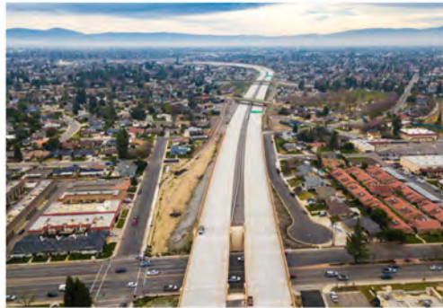
Centennial Mainline California Avenue undercrossing January 2024
