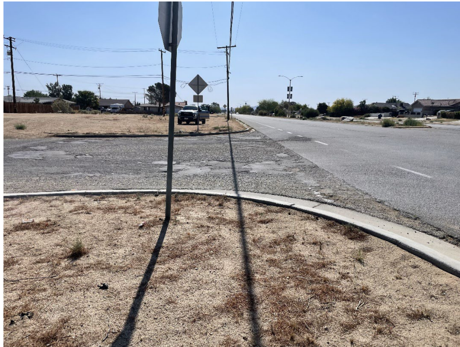
California City Blvd., East of Victor Way: No sidewalks, curb ramps, and damaged intersections.
