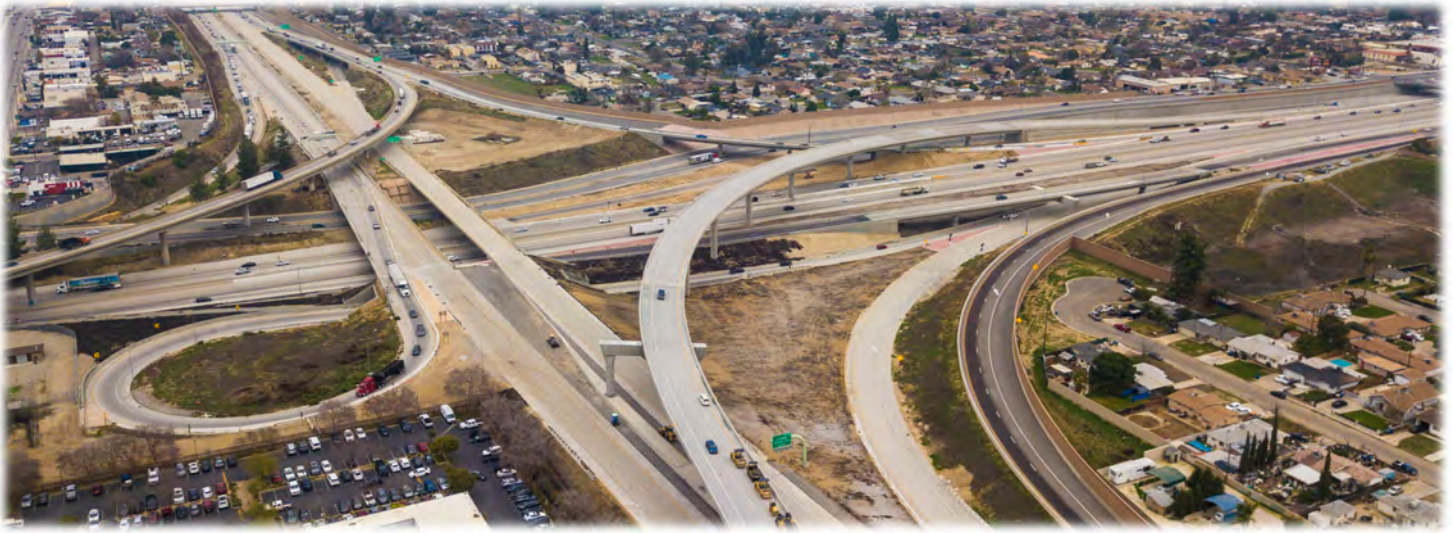
BAKERSFIELD FREEWAY CONNECTOR | LOOKING AT THE STATE ROUTE 58 AND 99 INTERCHANGE WHERE CONSTRUCTION EXTENDS THE 58 FREEWAY WEST AND BUILDS NEW RAMP CONNECTORS AND IMPROVES EXISTING RAMPS
