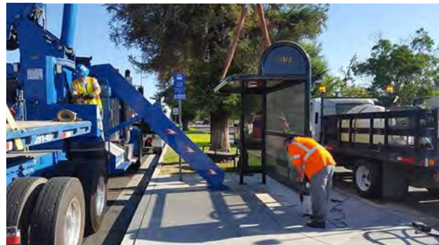
Installation of new bus stop
