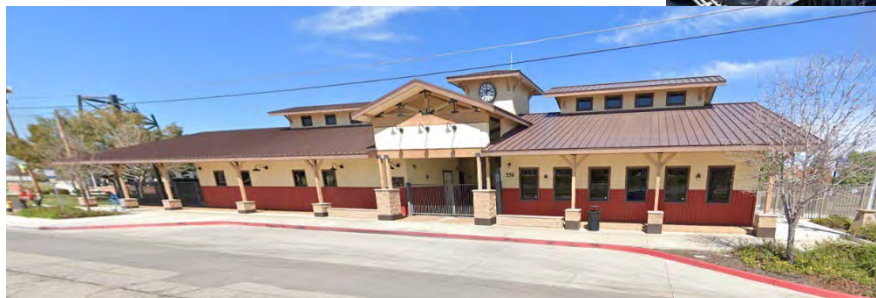
Constructed Taft Transit Center
