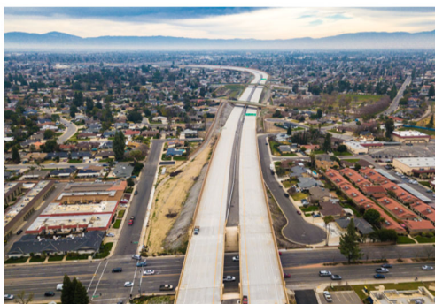
Centennial Mainline California Avenue undercrossing January 2024
