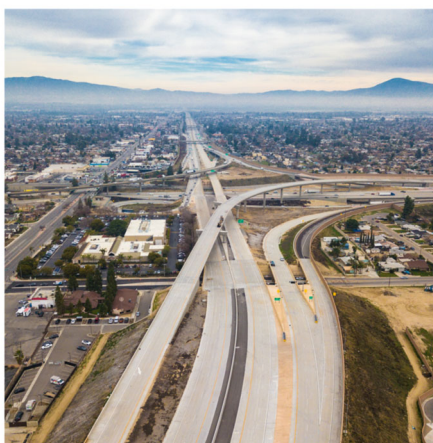
Centennial Mainline Real Road Bridges to various connector ramps. Looking east towards SR 99 & SR 58 January 2024
